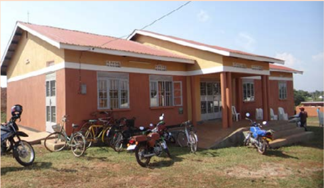
Tiira Town Council newly constructed administrative block, at Amagoro cell, Tiira ward, Tiira Town Council
