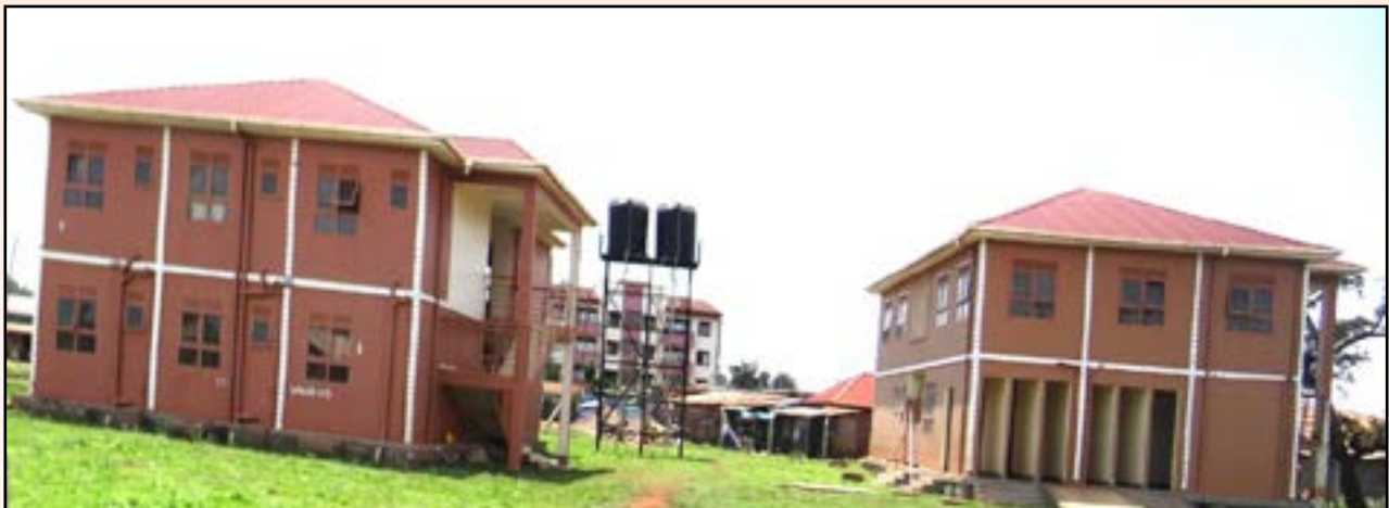
Some of the structures at the facility
