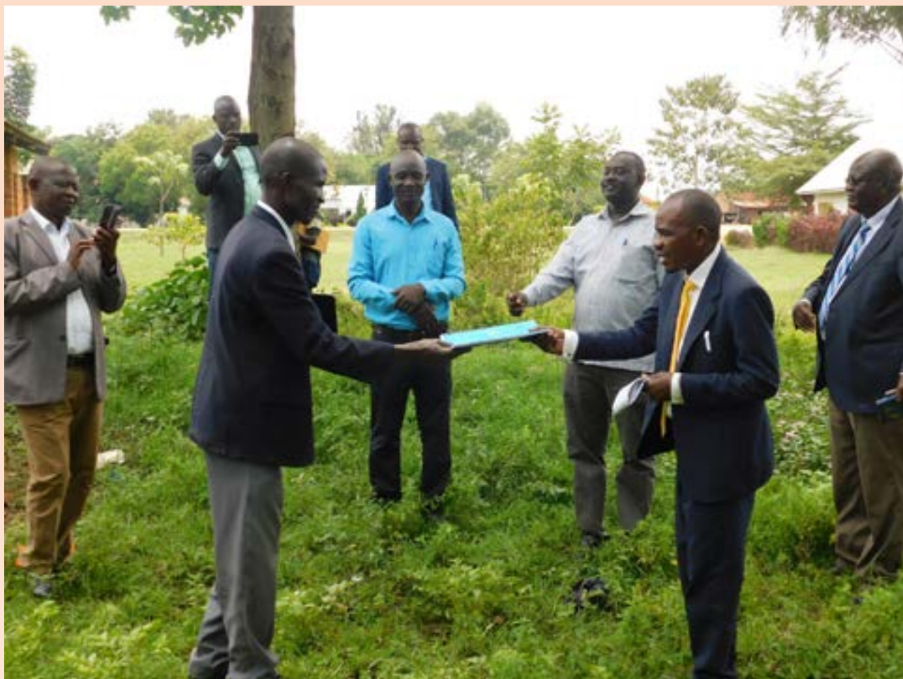
RDC Budaka Kimbugwe Husairu handing over a site for the construction of a 5-stance lined pit latrine at Sekulo Primary school to the contractor.
