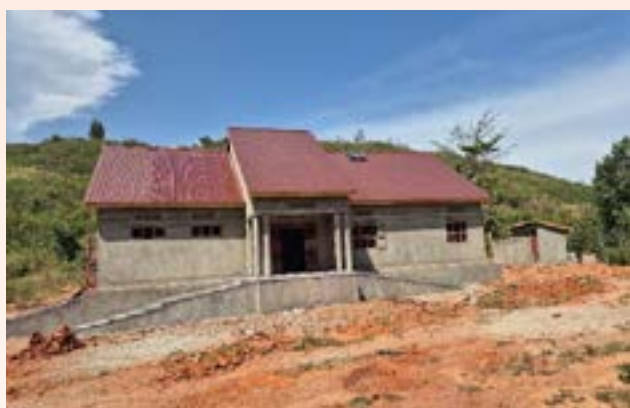
Lumino Administration Block under construction
