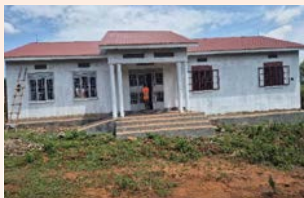
Tiira Town council Administration block under construction
