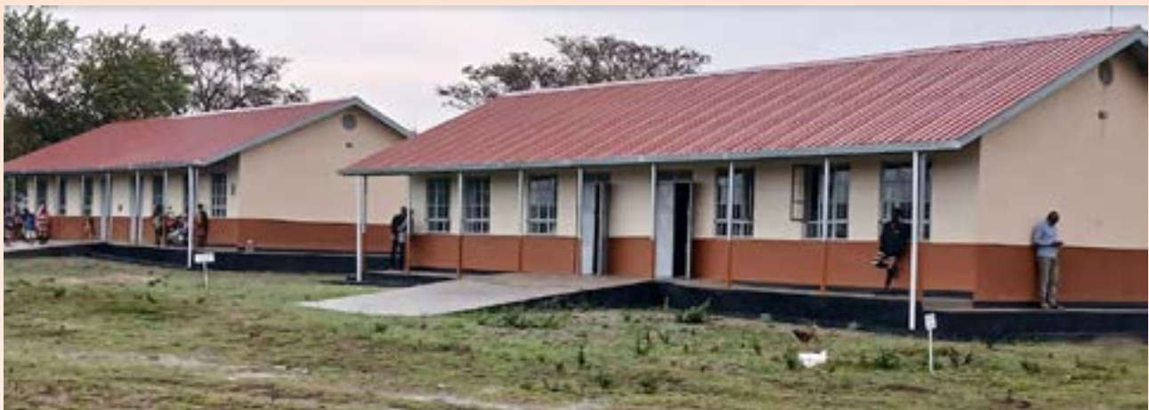
The newly constructed classroom blocks
