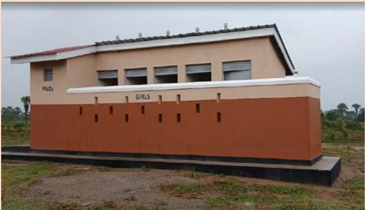
The school's washrooms
