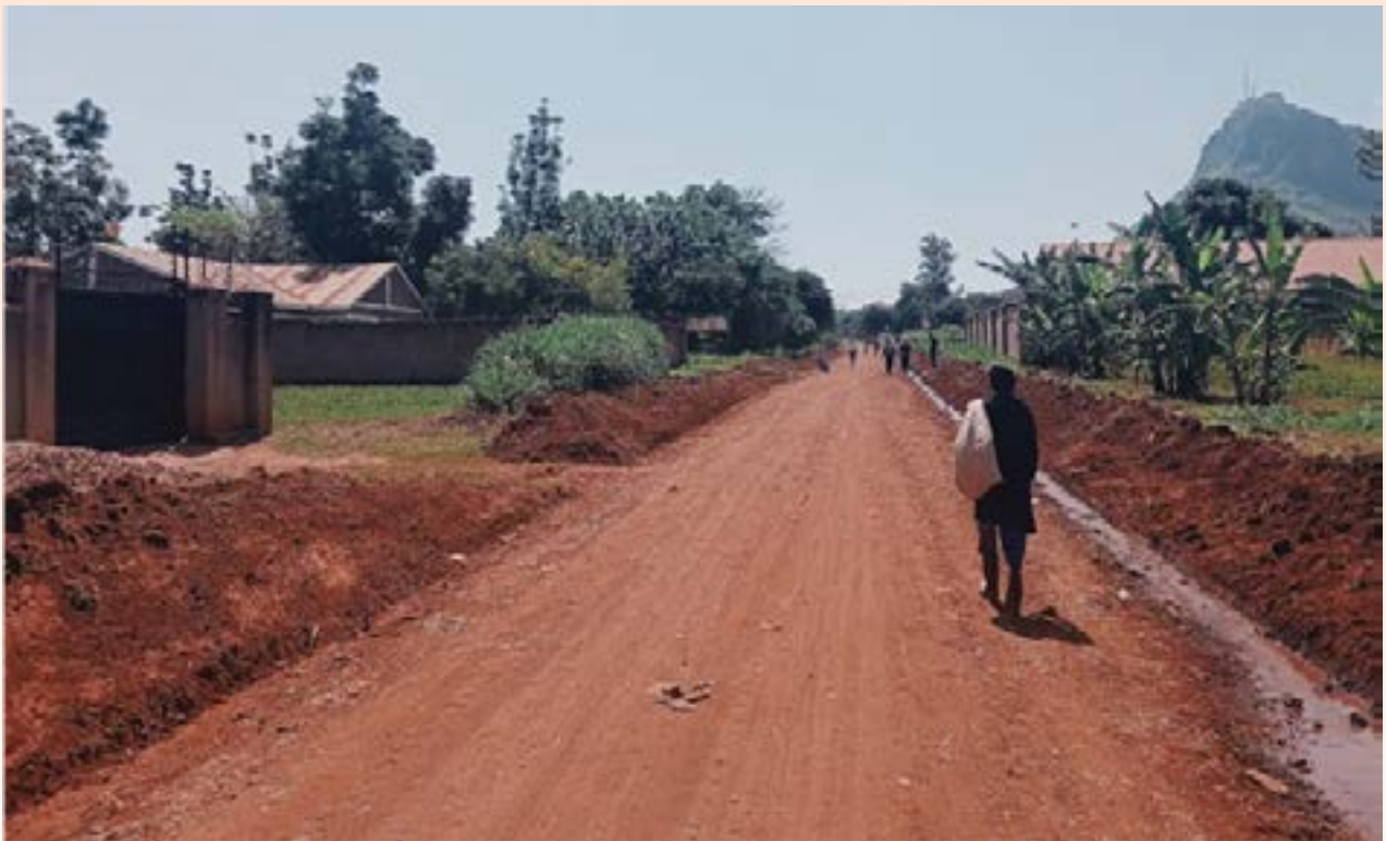
The road under construction
