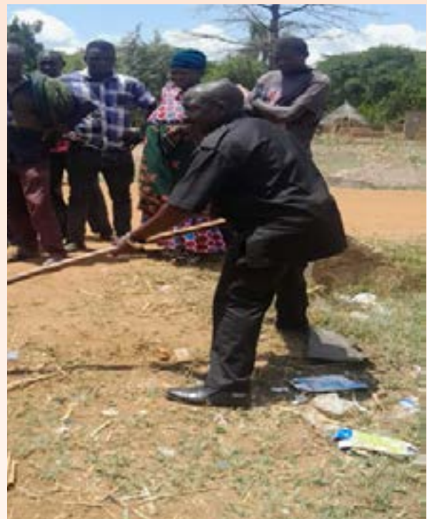
RDC Musiho Samuel launching Talisuna-Bukyera-Waibi-Kabusule a community access Road-6km
