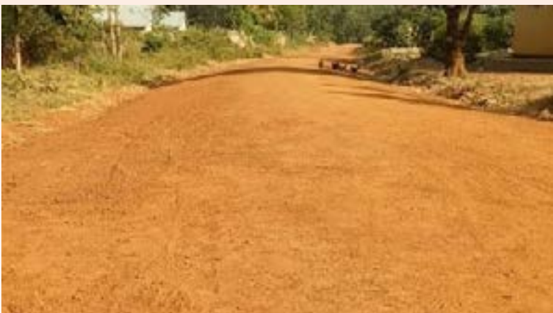
The new 13.2km Road From Kanyum Market to Kabelai
