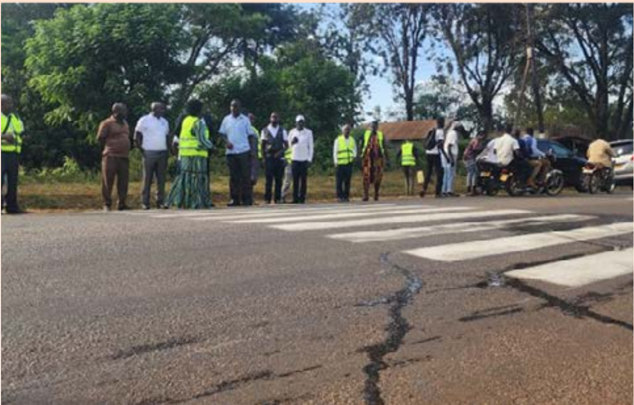
Stakeholders inspecting the Tororo-Mbale road
