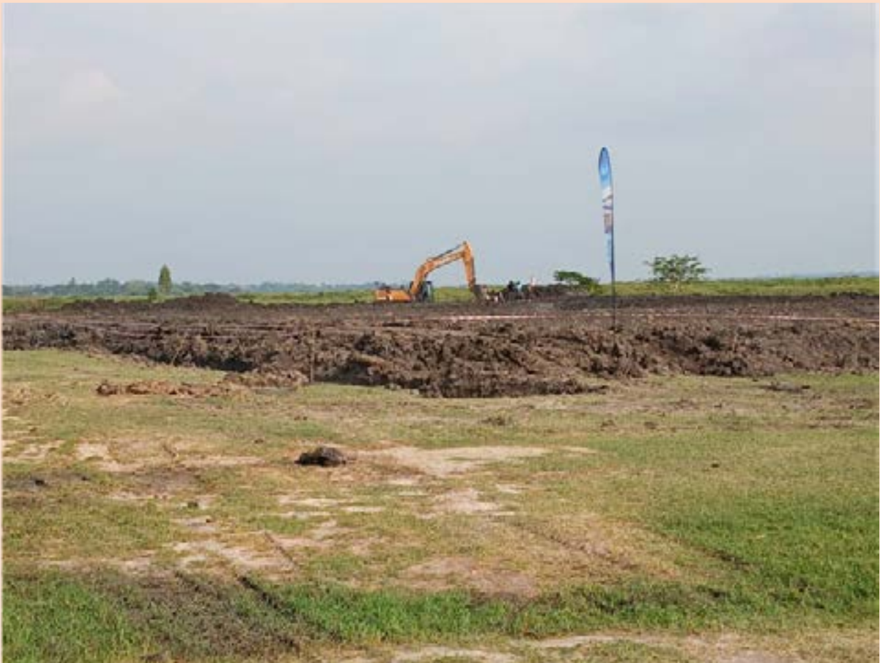
Digging of the fish ponds in progress
