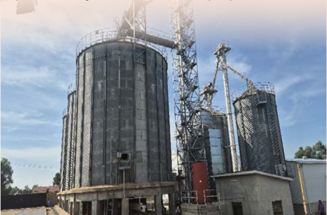
Some of the silos at the facility
